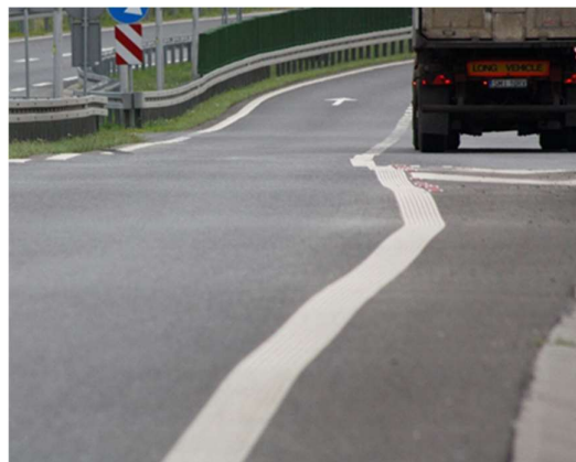
Figure 2. Uplift and settlement of the pavement surface caused by the use of ash addition in the construction of the road embankment layers (source: photo of M. Jastrzębska).
