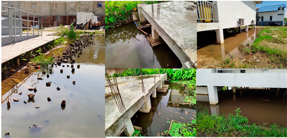
Figure 6. Foundation and Swamp Soil Environment.
