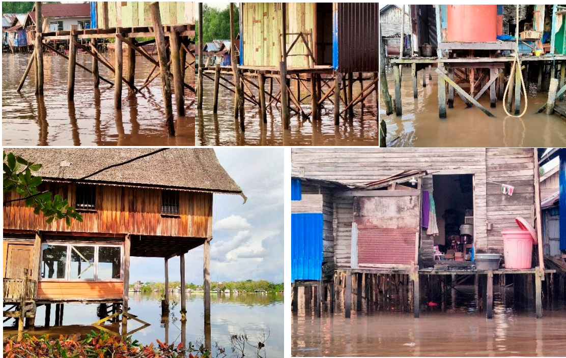
Figure 4. Foundations in Waterlogged Areas (River)
