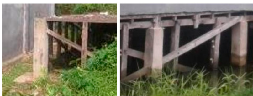
Figure 1. Combination of Wooden and Concrete Pile Foundations.
