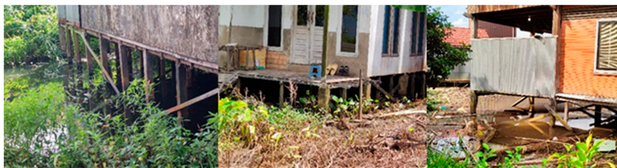
Figure 3. Foundations in swampland.
