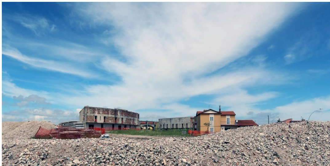
Figure 18. The social houses (IACP) in Bisaccia were designed by Aldo Loris Rossi immediately after the 1980 earthquake. The demolition phase (Photo from [49]).
