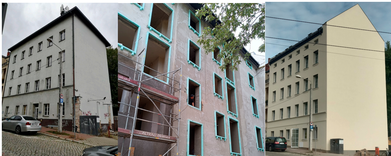
Figure 13. Case study building: before, during, and after renovation.
