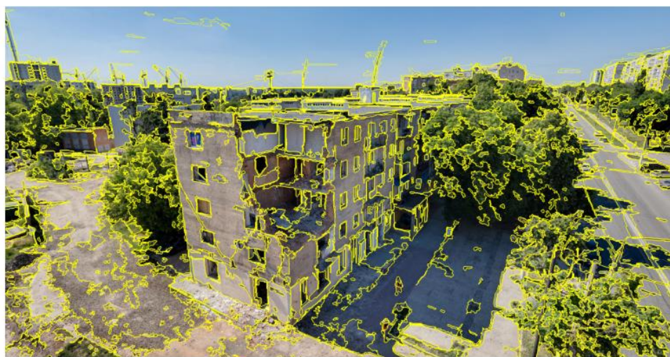
Figure 5. Output of Felzenszwalb segmentation (scale = 300, sigma = 0.9, min_size = 50) on a damaged building image. Yellow contours mark regions grouped by local color and texture similarity.
