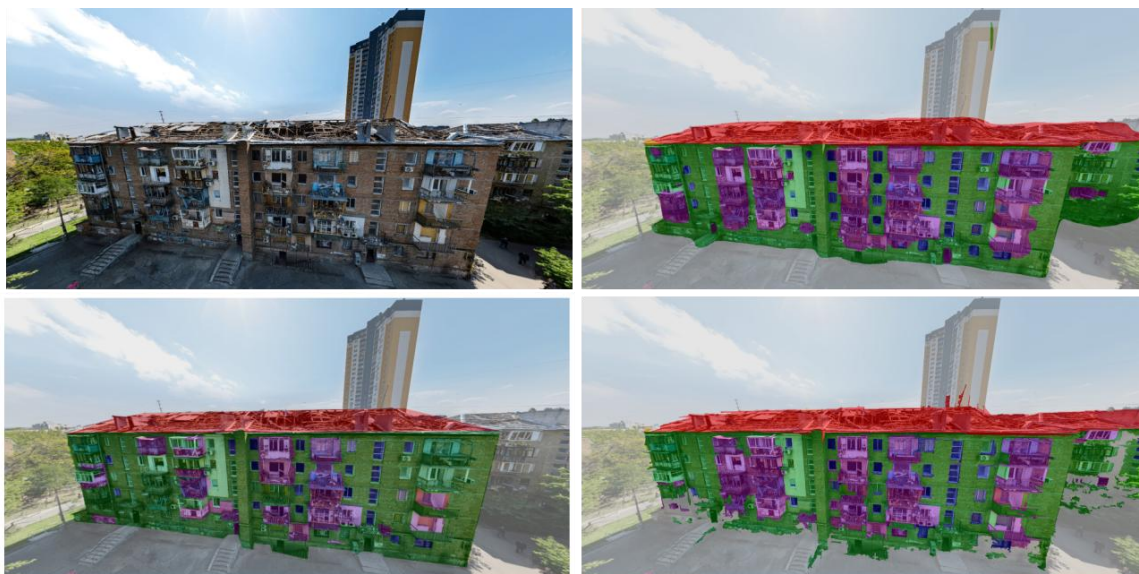
Figure 7. Effect of superpixels on the DINOv2-Emb model in the 6-class setup. Top left - original image, bottom left - ground-truth segmentation mask, top right - DINOv2 with embeddings, bottom right - DINOv2 with embeddings and superpixels applied. Color coding of classes: grey - Other, green - Building, purple - Damage, blue - Broken Window, orange - Roof, red - Damaged Roof.
