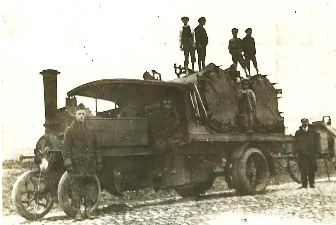
Figure 4. One of the ten mobile Foden-Thresh Mobile Sterilizers sent to Poland by the APRE in 1919. The Foden lorry was steam powered and supplied steam to the Thresh disinfector [22,61].
