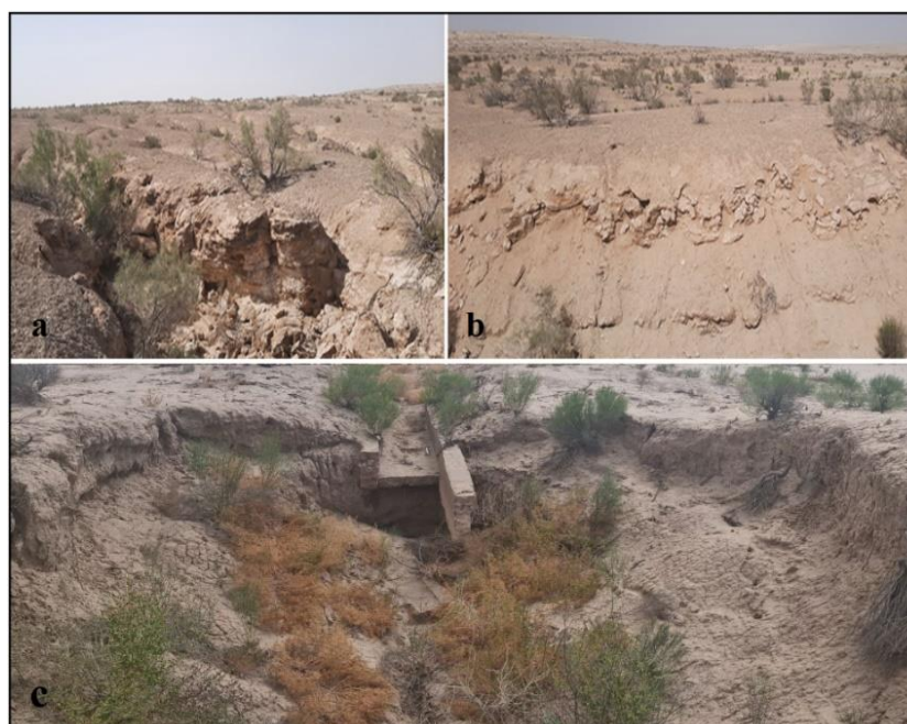
Figure 4. Erosion cuts a , b ) of ravines of gently sloping surfaces and c ) man-made ravine formation due to the malfunction of the guide water pipeline on the outskirts of the takyr of the Karakalpak Ustyurt (photo by K.M. Dzhaksymuratov , 2022, A.P. Akimova, 2024).
