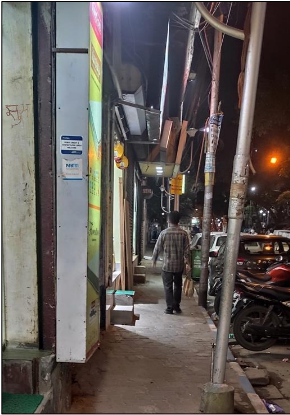
Figure 10: Street Lights inside footpath
