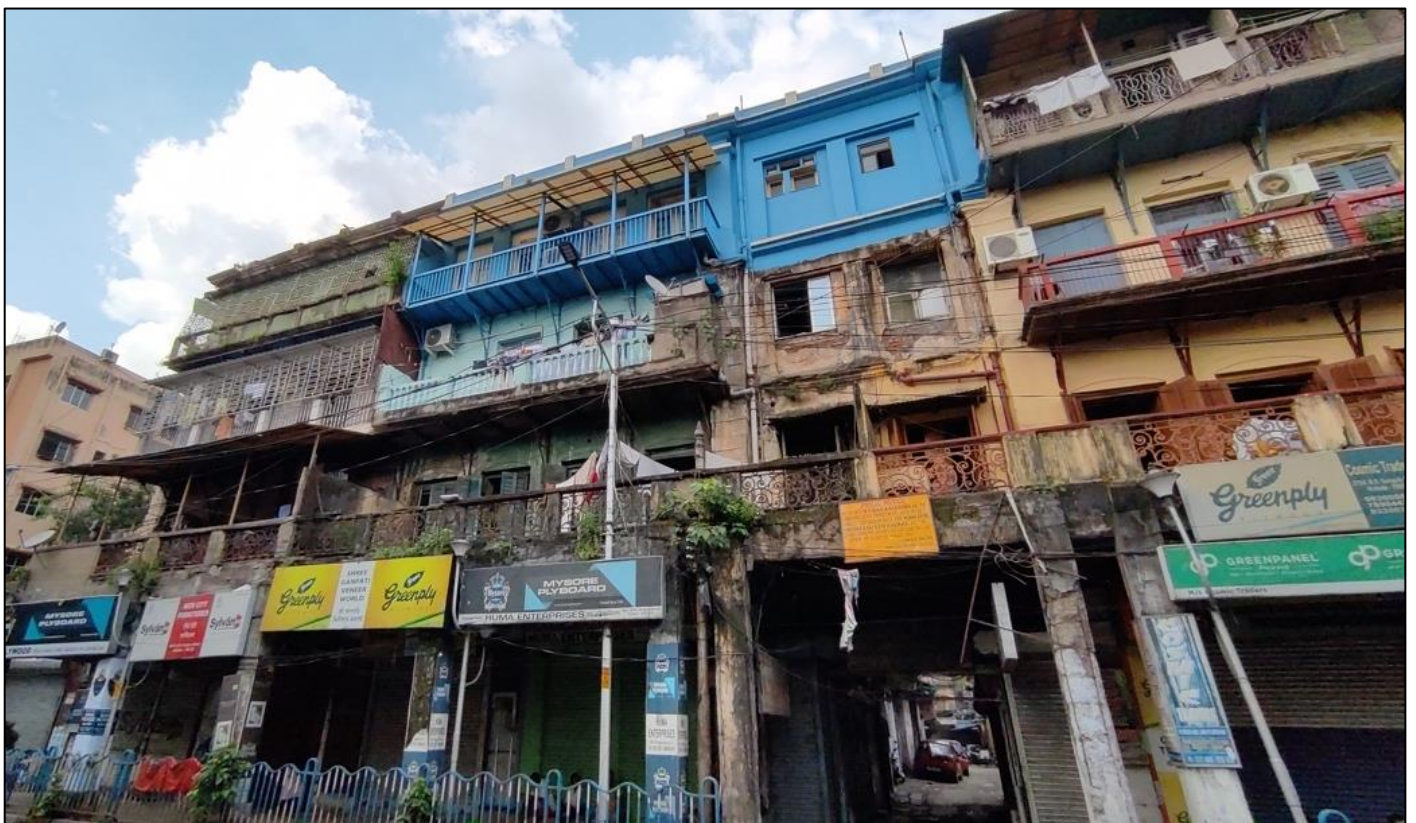
Figure 7: Mixed Use Buildings (Ground: Commercial; Upper Floors: Residential).
