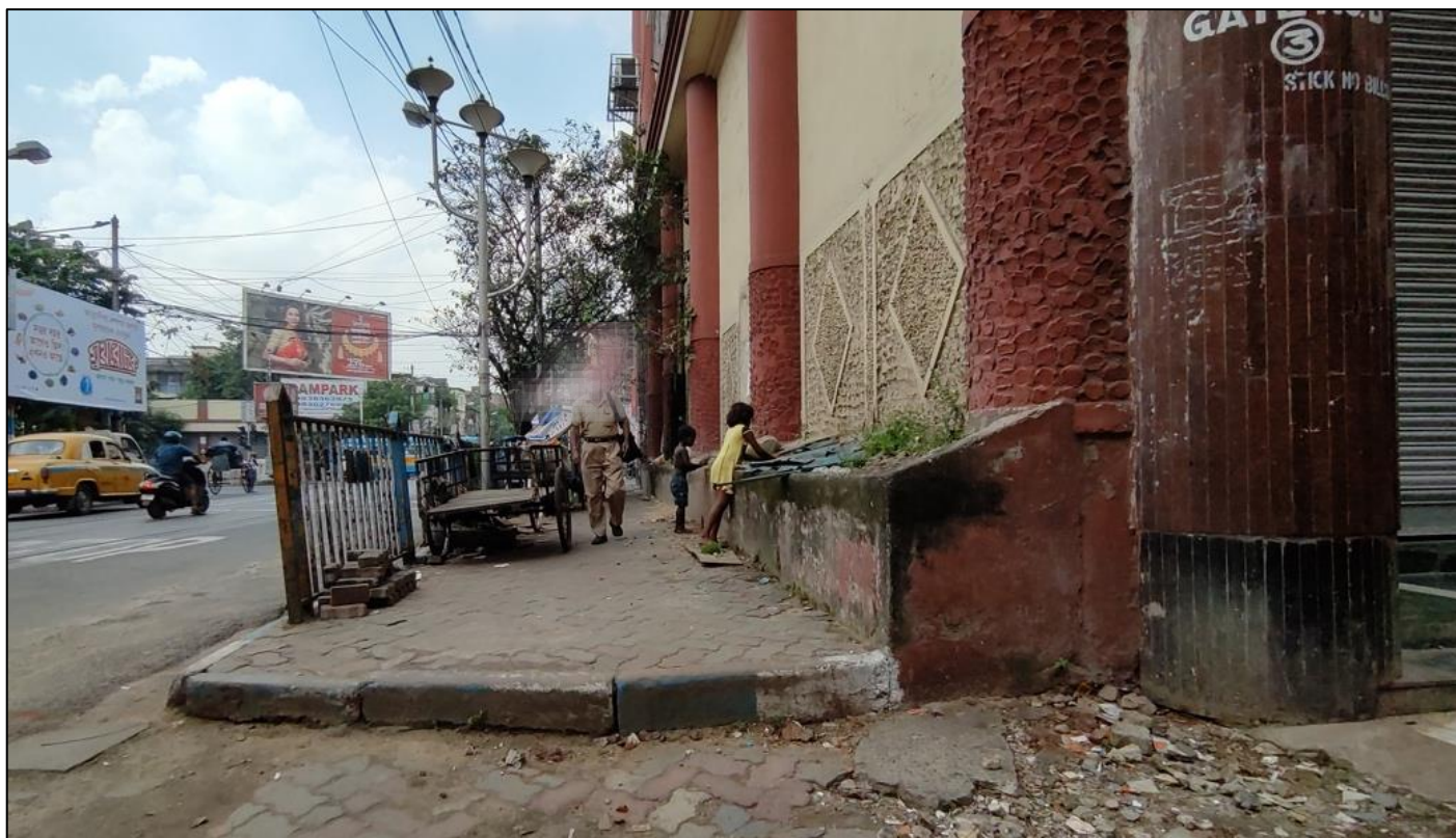
Figure 8: Footpath height improper for differently-abled people.
