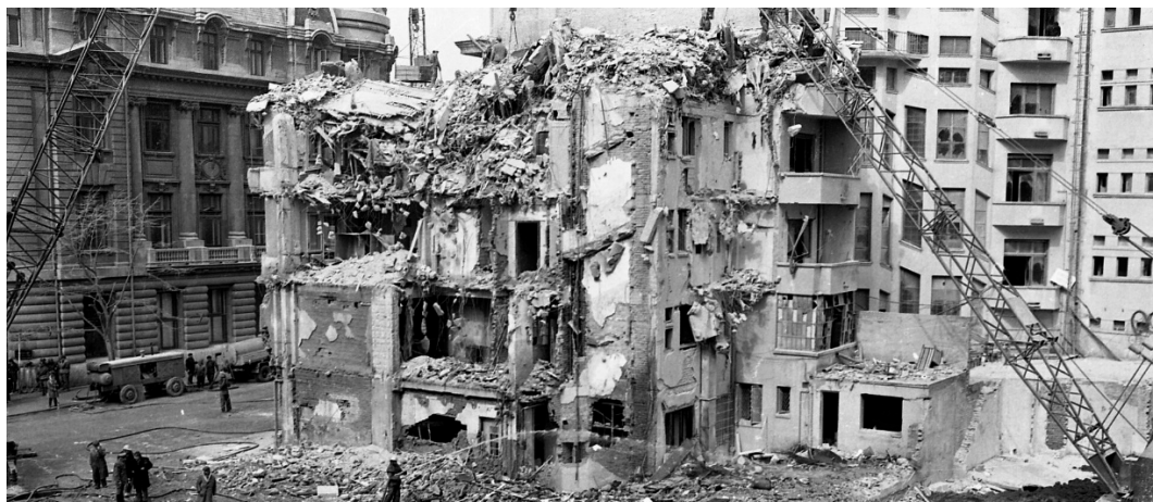
Figure 2. Partial collapse of reinforced concrete buildings in Bucharest during the 1977 Vrancea earthquake [34]
