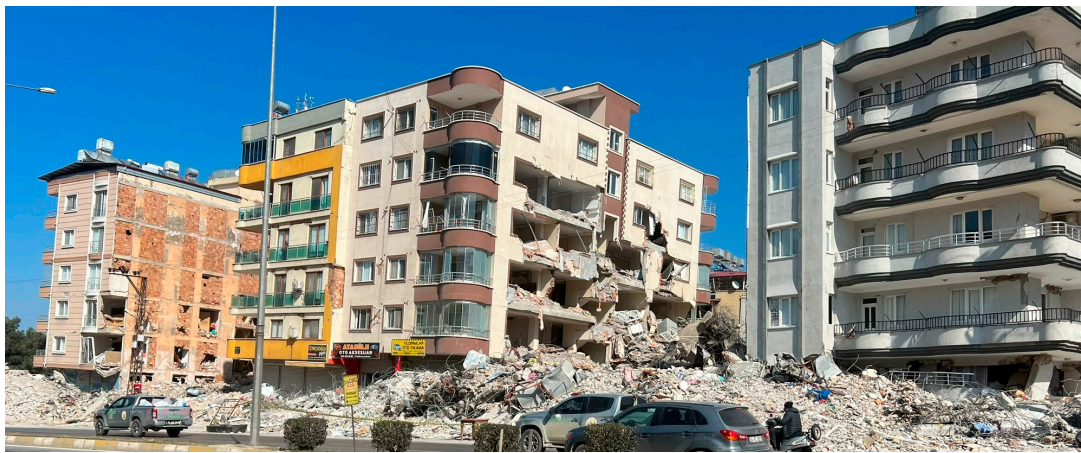
Figure 1. Partially collapsed reinforced concrete apartment buildings with masonry infill walls, Gaziantep, Türkiye, February 2023.
