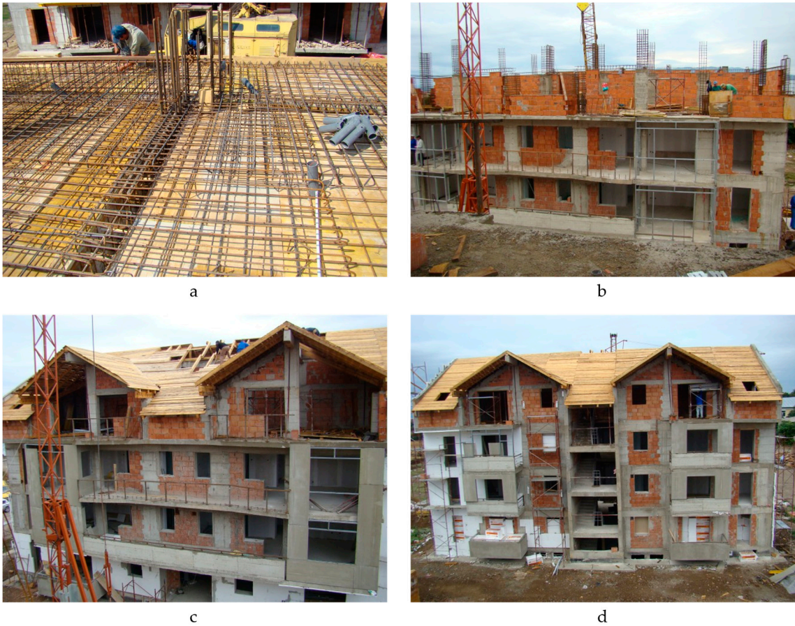
Figure 3. Construction stages of the RC frame building (a) - slab and beam reinforcement; (b), (c)- erection of RC frames and masonry infills; (d) - installation of the timber roof structure.
