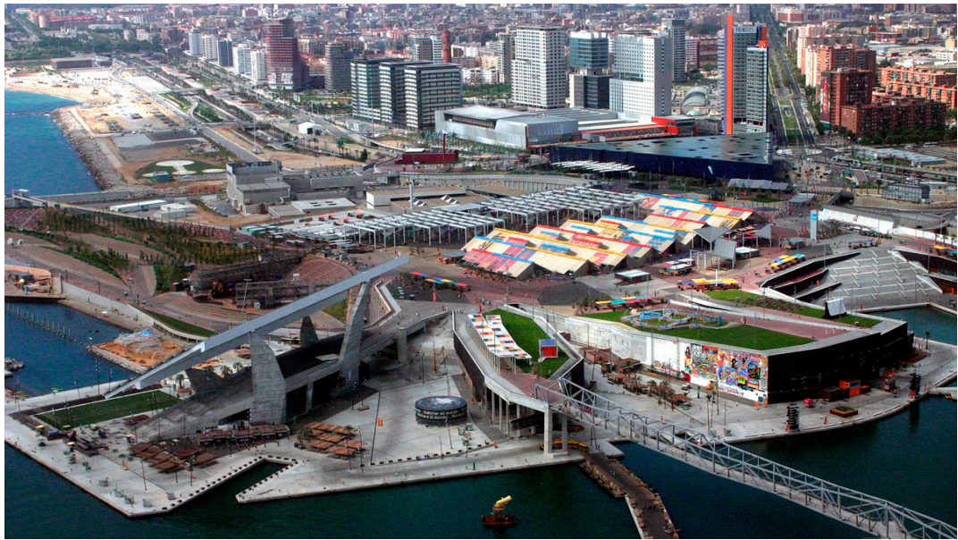
Figure 12. The urban complex of Diagonal Mar i el Front Marítim del Poblenou takes on the features of a major transformation project linked to a great event, even without fully integrating itself on a functional level into the city system (from Wikimedia Commons, licensed under CC BY 3.0).
