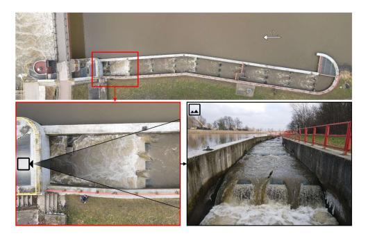
**Figure 3.** The impact of floating debris on the functionality of fish passes. The top image shows an aerial view of a fish pass, while the bottom images highlight areas of potential blockage and disturbance due to debris accumulation, which can impede fish migration and affect water flow dynamics (Wrocław, Poland).
