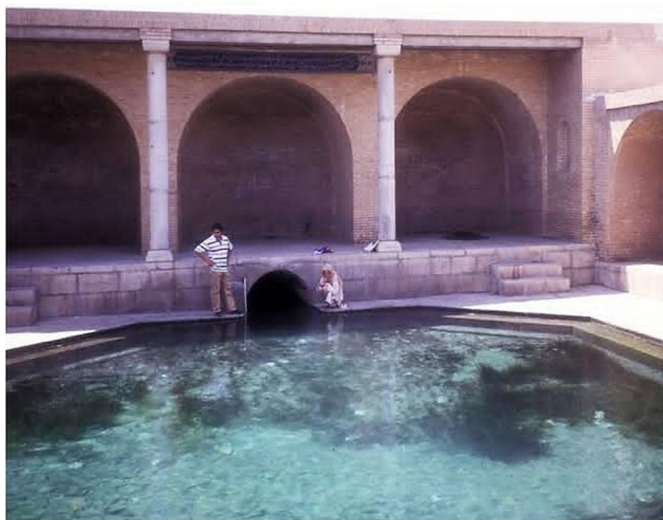
Figure 2. A Qanat's Outflow, Soleymaniyeh Fountain, Fin Garden, Kashan, Iran. With permission from: Torabzade, A. (2018). Traditional irrigation system of Sulaymaniyah spring in Fin of Kashan. Kashan Shenasi, 10(2), 158-171.
