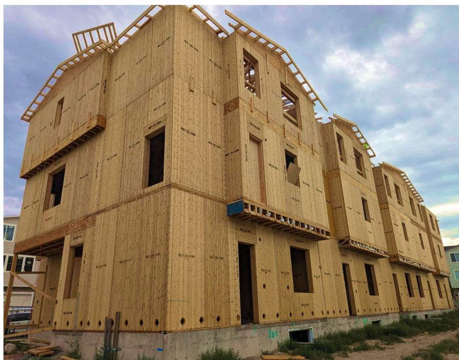
Figure 5. Three-story, building code compliant, vertical framing system using a composite of bamboo and wood (Source, BamCore).
