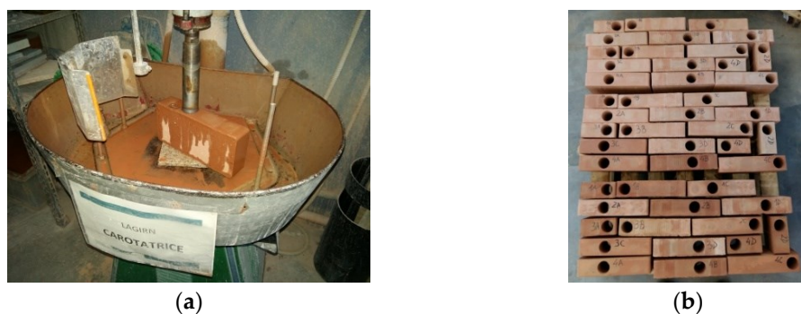
Figure 12. Preparatory stages for laying bricks: (a) Core drilling of a brick; (b) Drying of bricks after core drilling.
