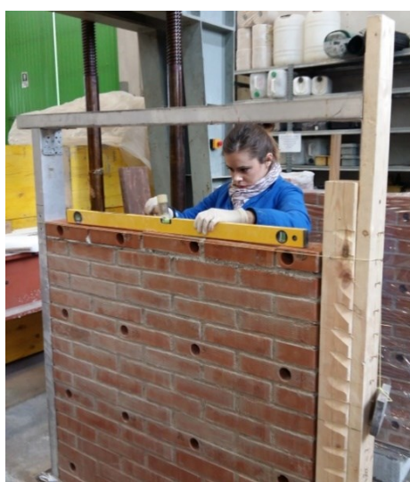
Figure 13. Equipment used for the correct laying of bricks.
