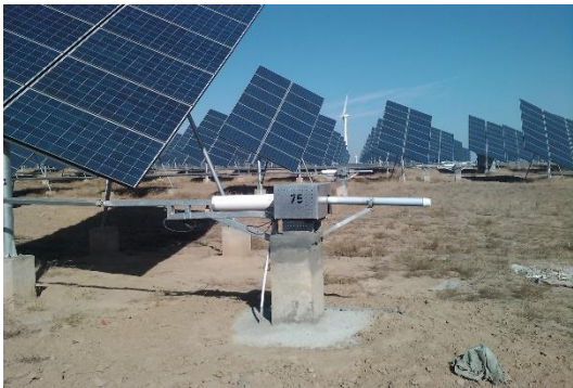
Figure 23. Linear actuator driving an array of polar axis solar trackers - China (Ningxia).
