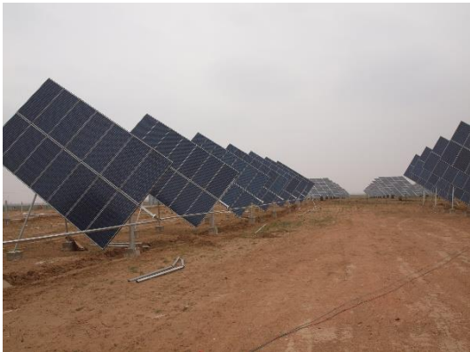
Figure 22. Array of polar axis trackers mechanically interconnected to a single driving unit.
