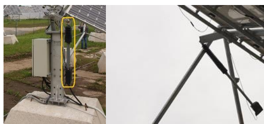
Figure 25. a, b Linear actuator at the bottom and top sides of the polar axis tracker.
