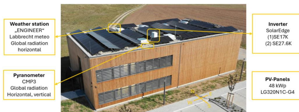
Figure 1. Solar and weather station installation on the Feuchtwangen campus.
