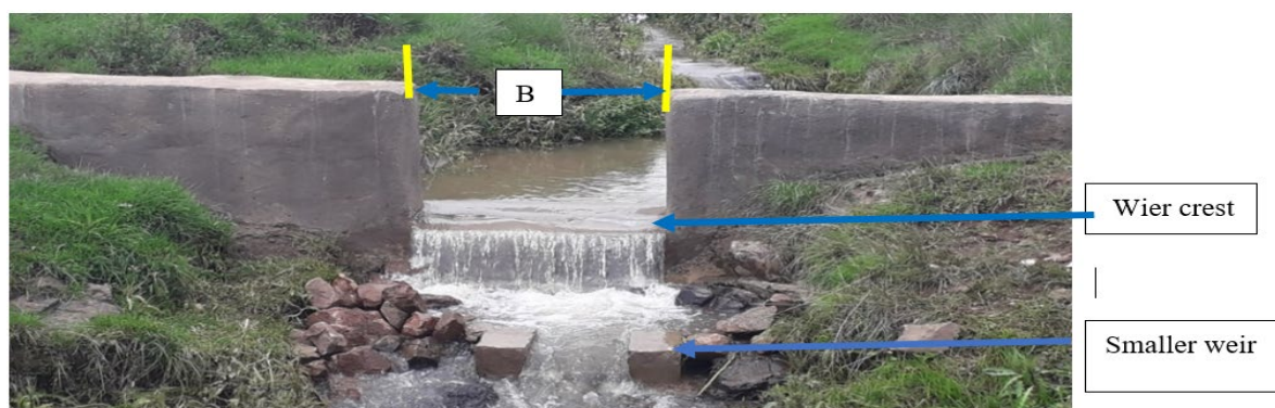
Figure 4. Stream flow measuring weir at the outlet of the research sites.
