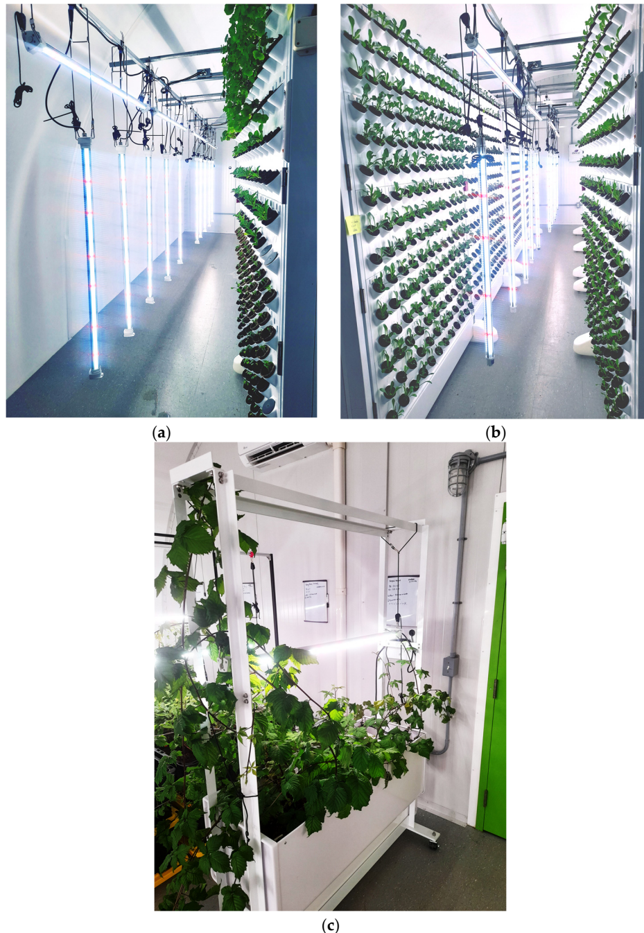
Figure 4. The location of lights and their applications inside the agrotunnel: (a) BGL180A on the side aisles; (b) BGL360A on the center aisles; (c) BGL180C on the grow bin.
