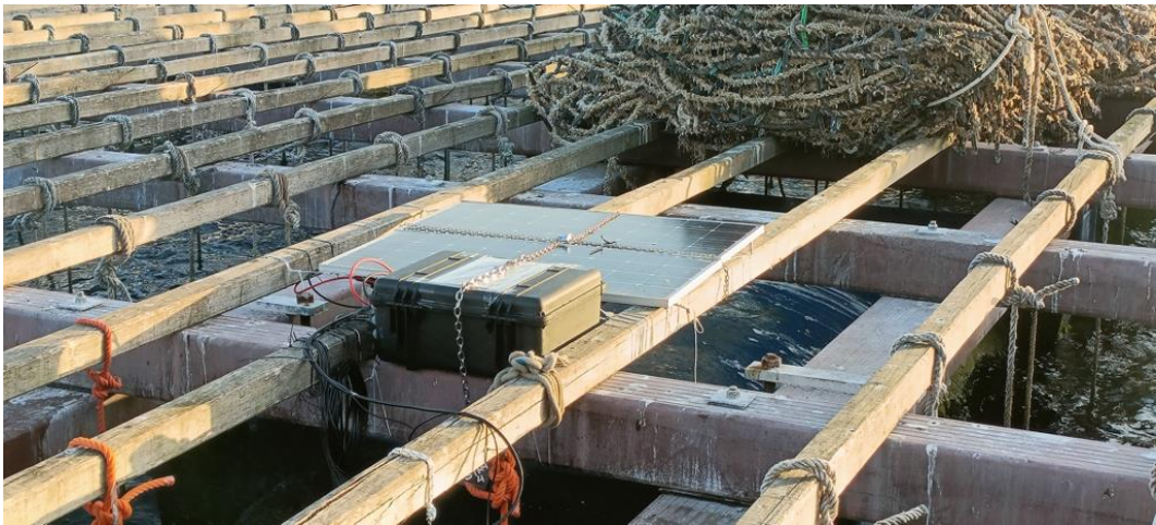
Figure 4. Top: electronics; Bottom: the Peli case with the electronics and the solar panels installed on the raft.
