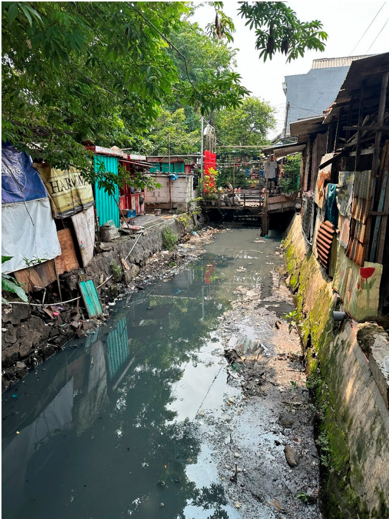
Figure 5. A view from Kampung Kue Rungkut showing its inadequate drainage conditions (photo credit: Author Iftekhar Ahmed).
