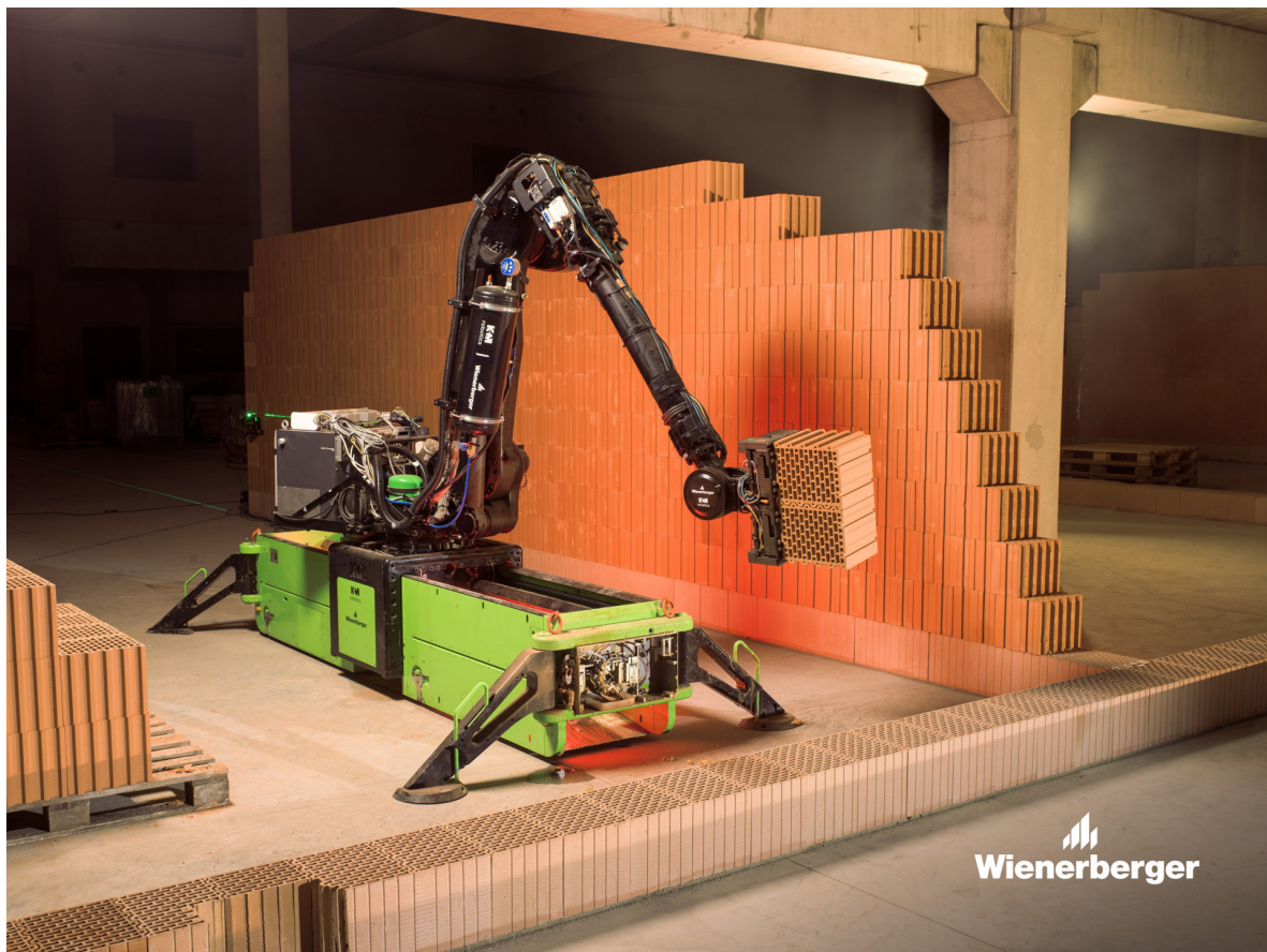
Figure 3. Wienerberger's WLTR masonry robot is an industrial robot on track placed in the construction site with a truck or a crane. It is aligned using a cross-line laser and monitors wall alignment with its sensors. It can pick up two bricks at a time and detect damaged ones, alerting the operator if misalignment occurs. The robot applies adhesive foam to the bricks before placing them with precision according to a virtual wall model. It communicates with an operator via a tablet and requires one supporting worker for tasks like supplying bricks and making adjustments. WLTR can move independently along the wall using a hydraulic lift and an electric pallet truck is included for floor movement. The system is very heavy and cumbersome for small-scale construction.
