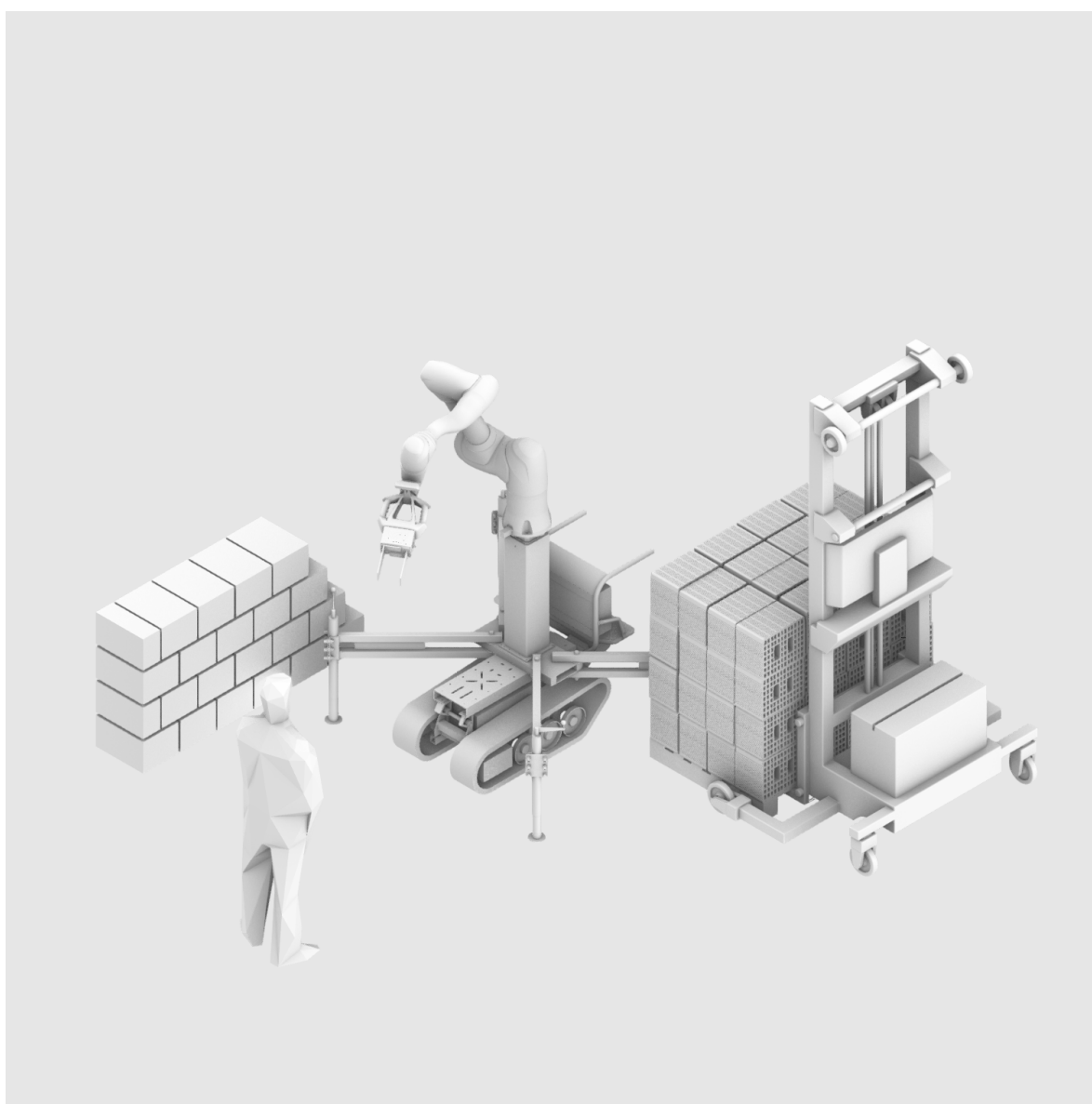
Figure 18. In the first phases of the construction process, the first clay block macro-row is being built with the clay block pallet on the ground and the lifting column retracted.
