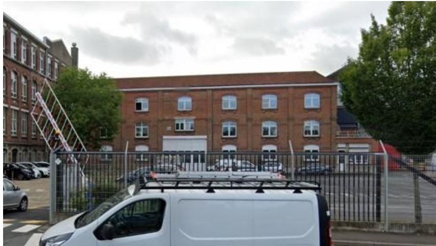
Figure 2. The building chosen for the case study.
