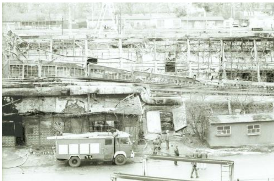
Figure 5. Burnt hall viewed from the shipyard side [19].
