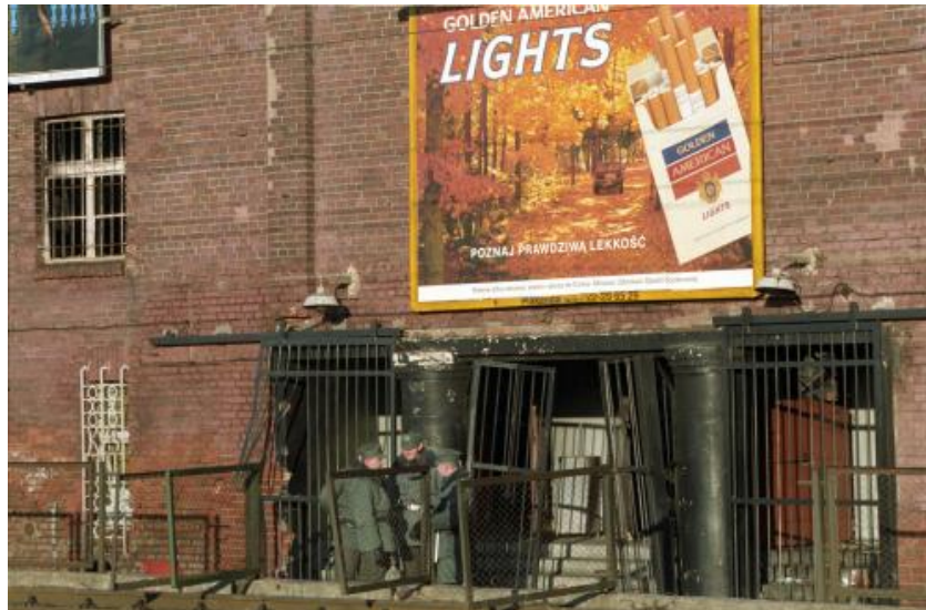
Figure 12. External emergency exit from the hall onto Jana z Kolna street. The photo shows the results of the rescue teams' efforts: bent grating bars and fence sections removed from the tram line (PAP/Alamy Stock Photo).
