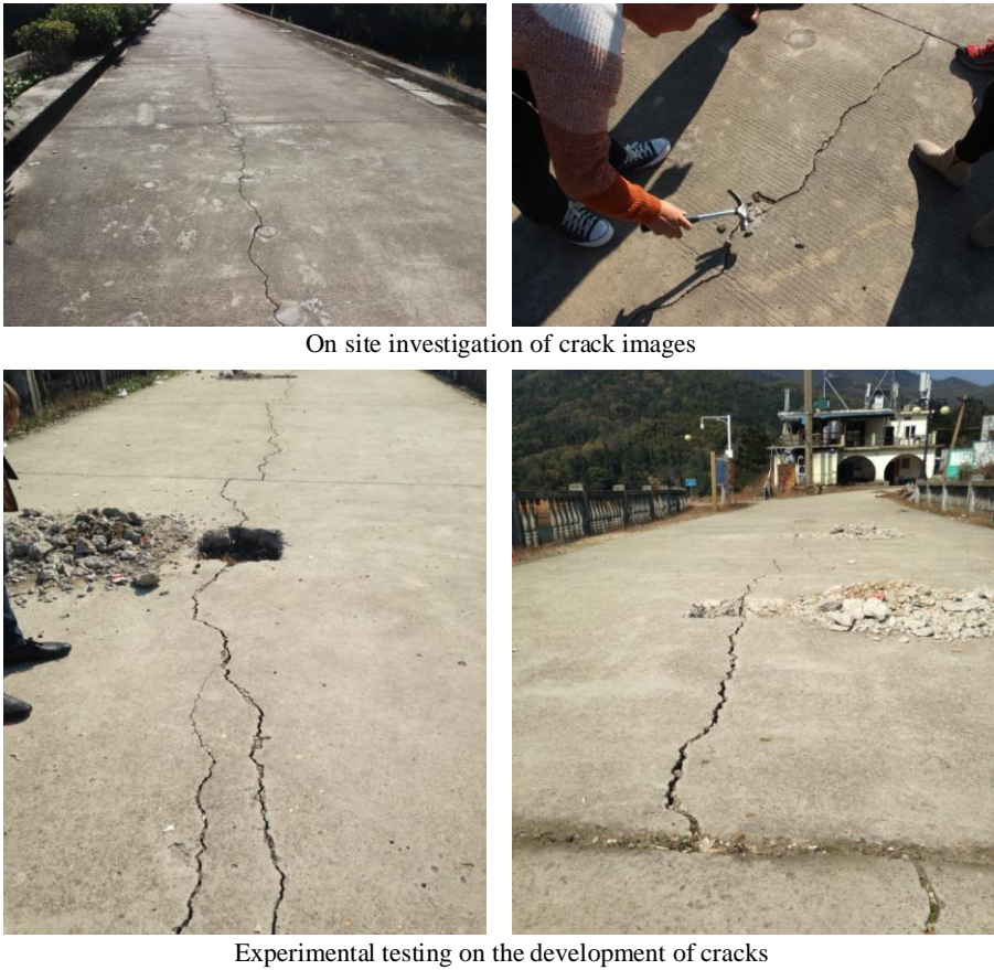
Figure 2. Crack hazard investigation in small-scale reservoir engineering.
