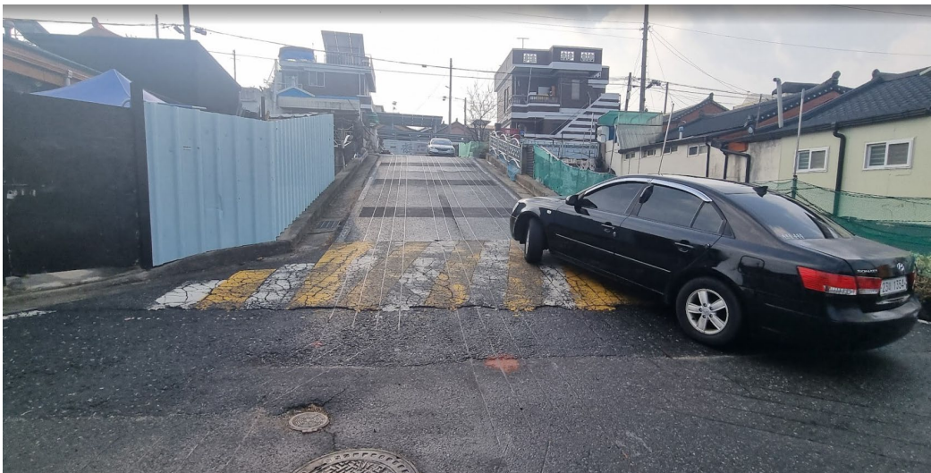
Figure 3. Heated road surface with embedded RHS coils at Namgyeong-maeul Road (Nov 4, 2024).
