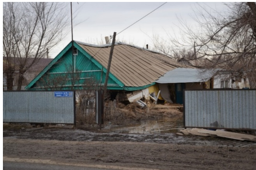
(a) Destroyed houses in the village of Kobda
