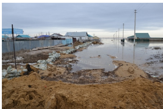
(c) Flooding in the village of Kobda
