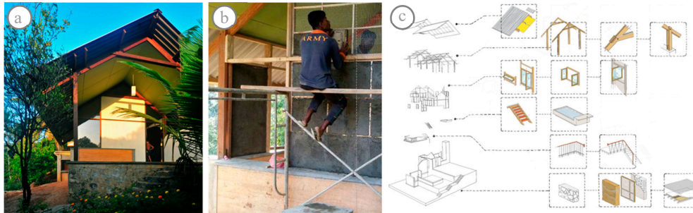
Figure 6. (a) Wakwella house; (b) Soldier-labour; (c) Kit of part building system for flexibility and transferability.
