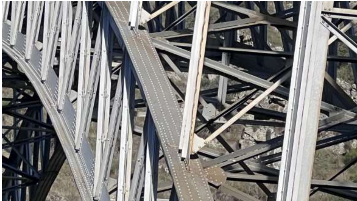
Figure 9. Examples of upright supports on the arch, using gusset plates fastened with bolts, on the upstream side (photograph by the author, taken with a drone).
