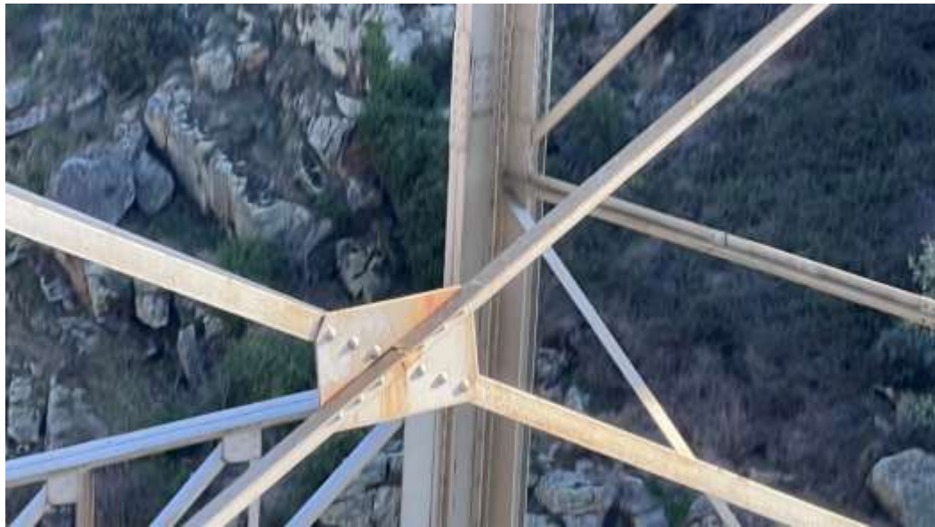
Figure 16. Localized corrosion on one of the braces of the sheet pile walls at the western end of the bridge, upstream side (photograph by the author, taken with a drone).
