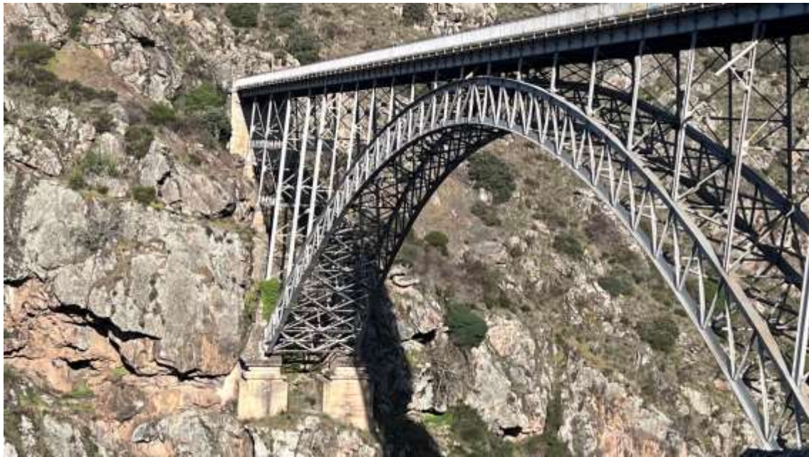
Figure 7. Partial view of the bridge from the southern side (upstream side), showing the main arch and, in the background, the second abutment with its corresponding support trestles (photograph by the author, taken with a drone).
