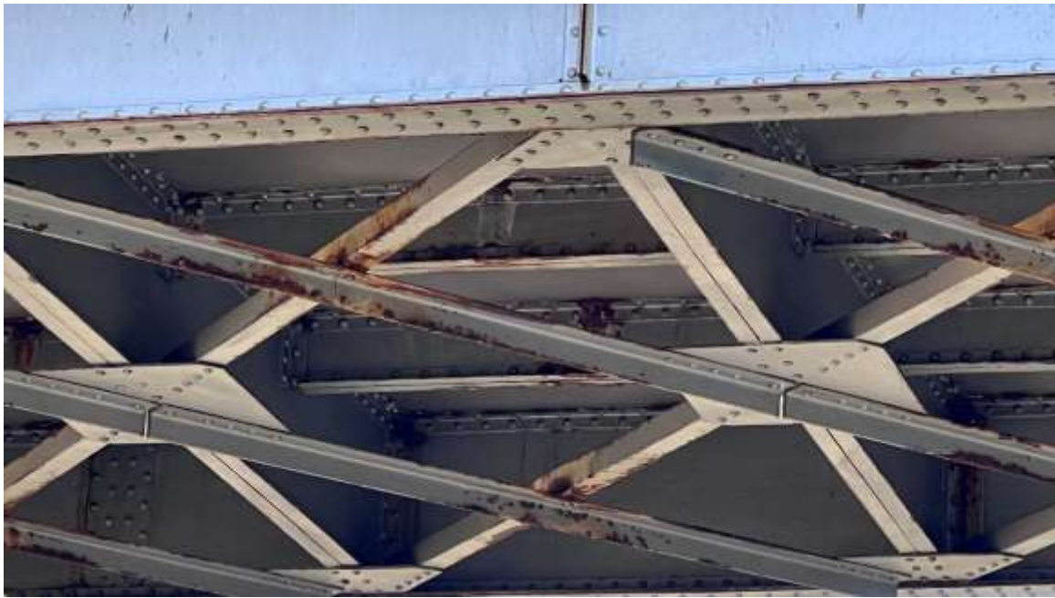
Figure 22. Detailed view of a deck section with localized corrosion on several elements (photograph by the author, taken with a drone).
