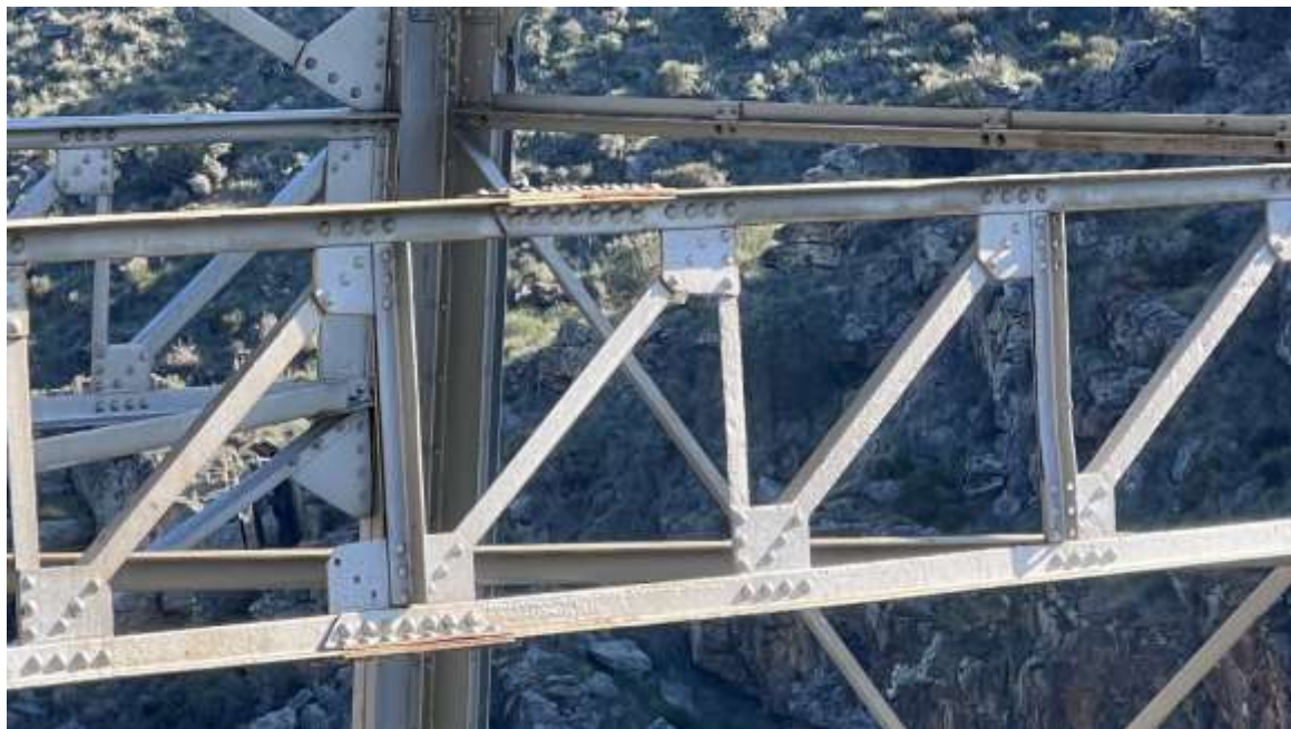
Figure 19. Detailed view of an arch section with localized corrosion at connection points (photograph by the author, taken with a drone).
