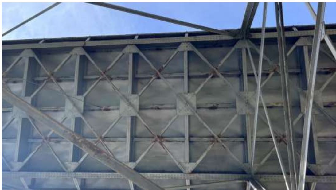
Figure 21. Bottom view of a deck section, showing numerous elements with localized corrosion symptoms (photograph by the author, taken with a drone).
