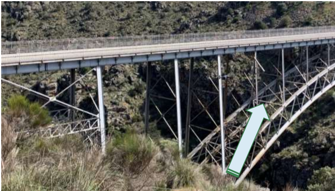
Figure 11. Multirotor drone approaching the Requejo Bridge to inspect the trestles of the second abutment from the upstream side (photograph by the author).
