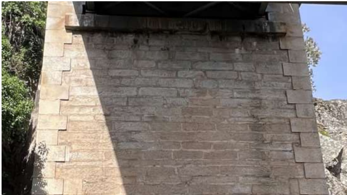
Figure 12. Wall of the second abutment with runoff water traces (photograph by the author, taken with a drone).
