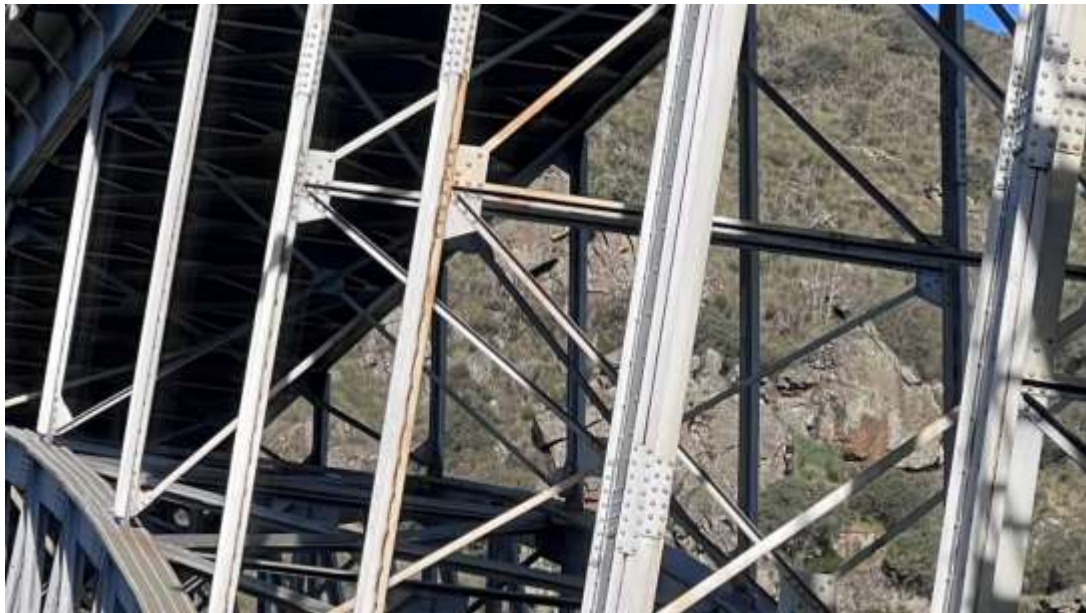
Figure 20. Detail of corrosion on one of the uprights over the arch (photograph by the author, taken with a drone).
