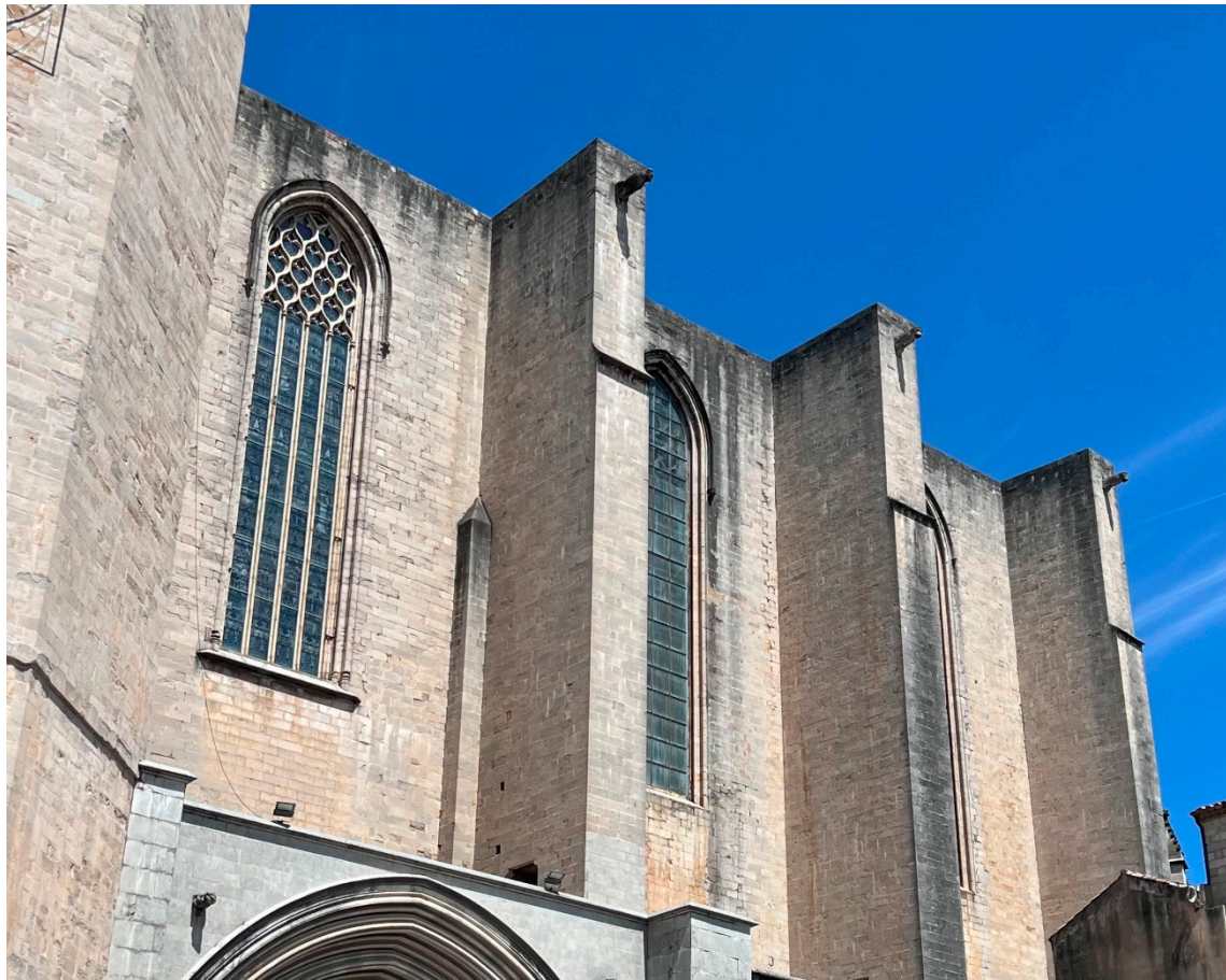
Figure 5. View of the southern façade of the Cathedral, showing the existing buttresses. The Romanesque tower is partially visible on the left and acts as the first buttress (photograph by the author).
