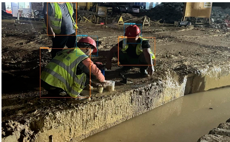
Figure 11. Night-time construction inspection results.
