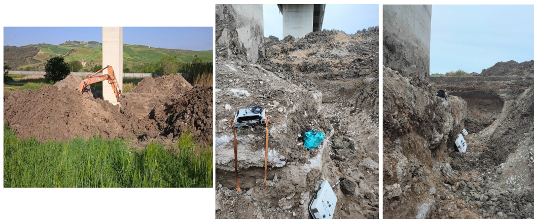
Figure 2. Excavation of the foundation for drainage maintenance and acquisition steps with the antennas, control unit, connection cable reel.
