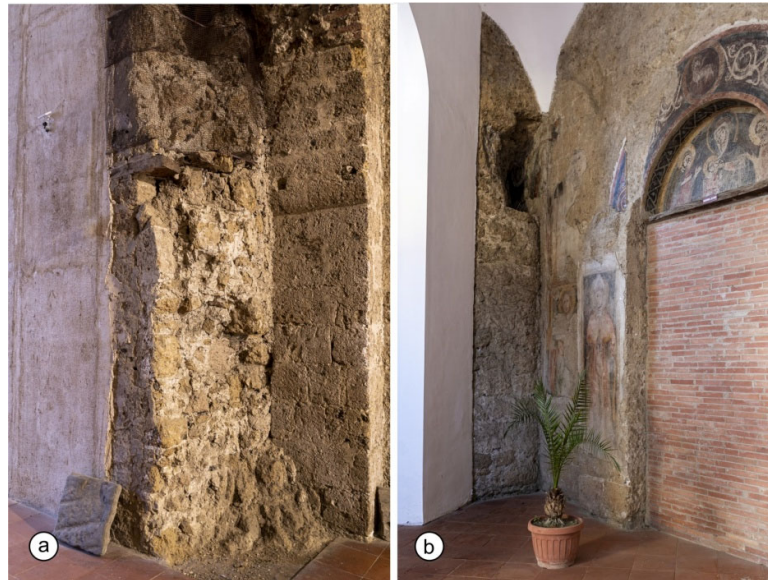
Figure 7. Examples of walls built with (a) technique “a cantieri” and (b) with technique “a bozzette”.
