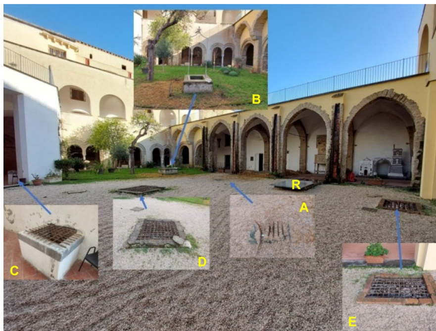
Figure 10. View of the cloister courtyard with location of the accesses to the underlying hypogea: R-ramp, A-E well.
