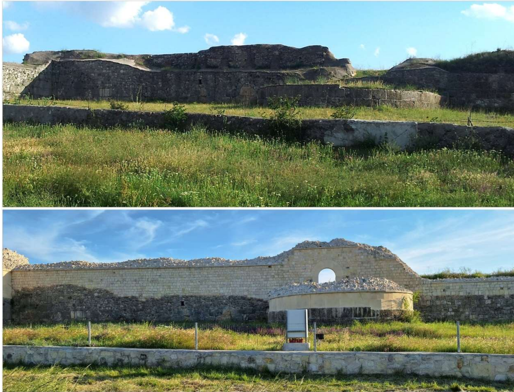
Figure 5. Curtain F and Tower 5, before and after the last intervention [32] (Dumitru M., 2013 – top; Florin Anghel, 2023 - bottom). The medieval fortification wall can be observed on top of the Roman curtain (top); protected with cement cap and consolidated with improvised buttresses soon after the excavation, it was probably sectioned by the early excavators with the purpose to investigate the tower entrance. The recent intervention replaced the medieval curtain with by heightening the Roman wall, completely annulling the existence of the former on this segment – where it was best preserved (!) The green cap visible on curtains E and D is probably what remained visible from the original structure, which was probably hidden behind the face of the new wall.
