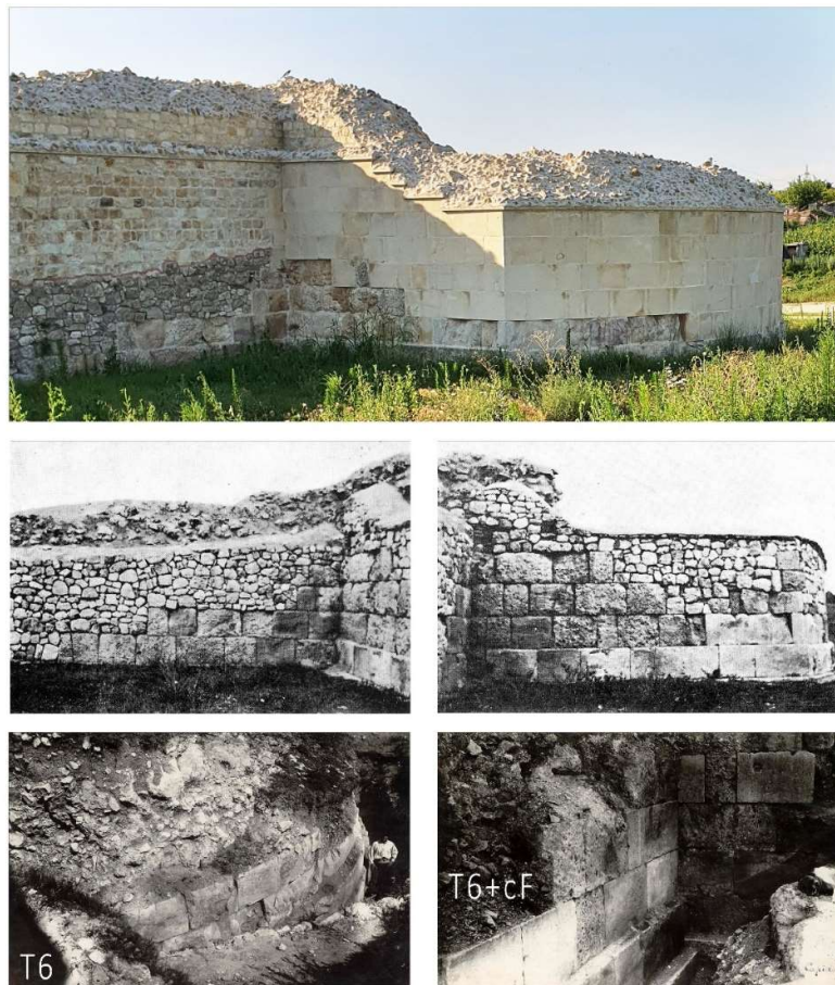
Figure 3. Curtain G and Tower 6 after the recent intervention (top) [32] (Lana Mariana Nicoleta, 2021), and before, with the additions of the 20 th c. (middle) [29] (figs. 33-4); it is obvious that the irregular parament of small blocks represents the latter, if compared to photographs upon the tower's discovery (bottom) [31]. Therefore, the red line in the recent intervention delimitates it from the previous one of the 20 th c., not from the authentic structure, as the doctrine says, thus misleading the reader. In fact, even if the red line would be missing, the most intuitive interpretation would be the same because of the high contrast, both in colour and stereotomy, between the recently added material and the others. Notice also the reconstruction of the “medieval” wall on top of the heightened Roman fortification (top); as for the photos in the middle (taken after the interventions of the half 20 th c.), it is difficult to assess whether on top of the curtains there are fragments from the emplecton of the same wall, or the remains of the medieval fortification, or simply rubble.
