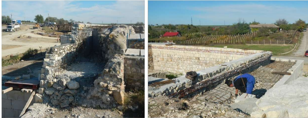
Figure 4. Reinforced concrete used for the so-called consolidation of the original 2.5-2.7 m wide Roman fortification walls (Alexandra Teodor, Oct. 2015).
