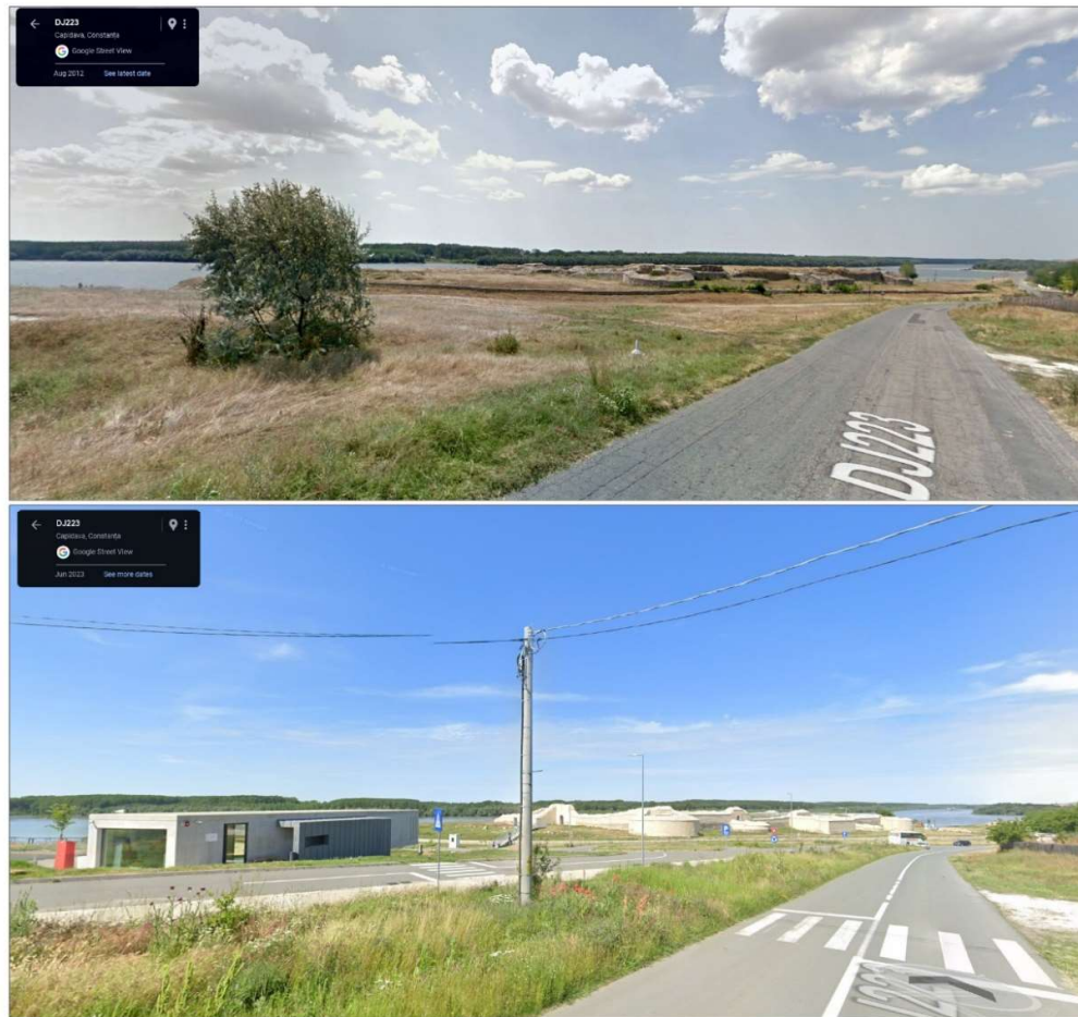
Figure 8. The descending view towards the fortification, coming from south. Before the intervention, in 2012 (top), and after, in 2023 (bottom) [32]. Notice also the new information centre / museum in the foreground.
