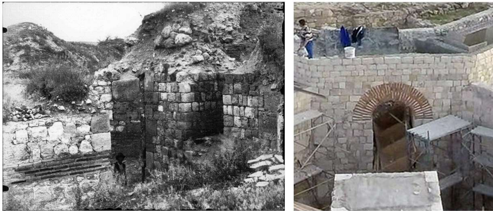
Figure 7. Tower 2, interior, after the excavation [31] and after the last intervention [43].
