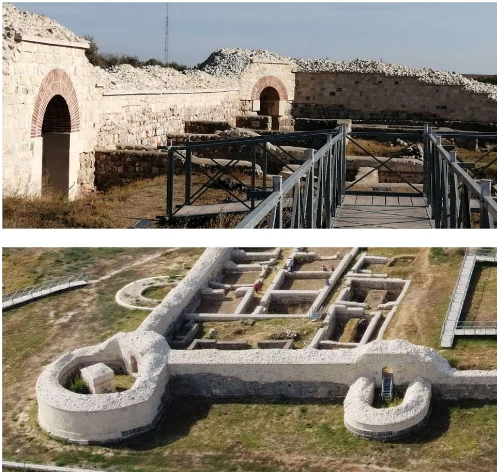
Figure 6. Towers 5 and 6, intra muros view (top) [32] (Tiberiu Costin, 2022) and aerial view (bottom) [32] (Cosmin Bodeanu, 2021). Notice the brick arches of the entrances towards intra muros , versus brick arch (T6) and stone arch (T5) towards the interiors of the towers. Both solutions are misleading since no relevant data was preserved for the elevations at this level, while the use of both techniques indicates some sort of certainty regarding distinct phases.
