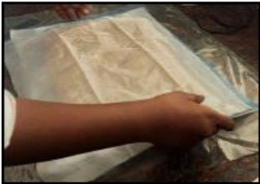
Figure 7. Placement of peel ply fabric over the resin -impregnated fiber mat.
