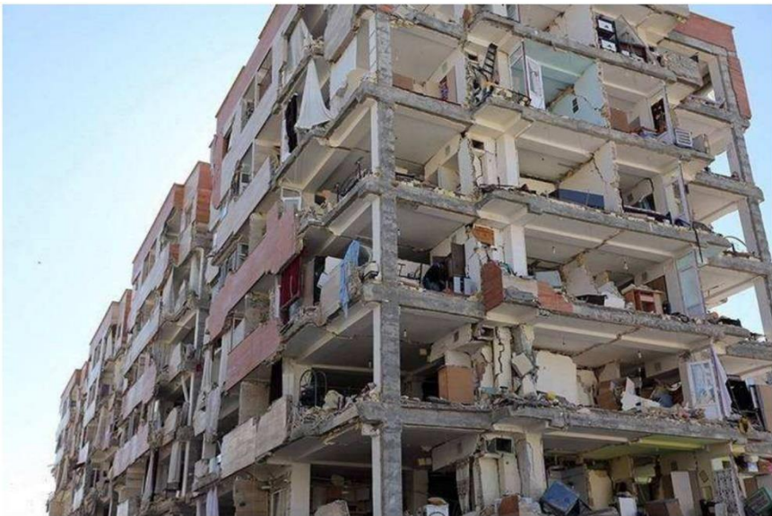
Figure 2. Damages to exterior walls in Life Safety limit state [4].
