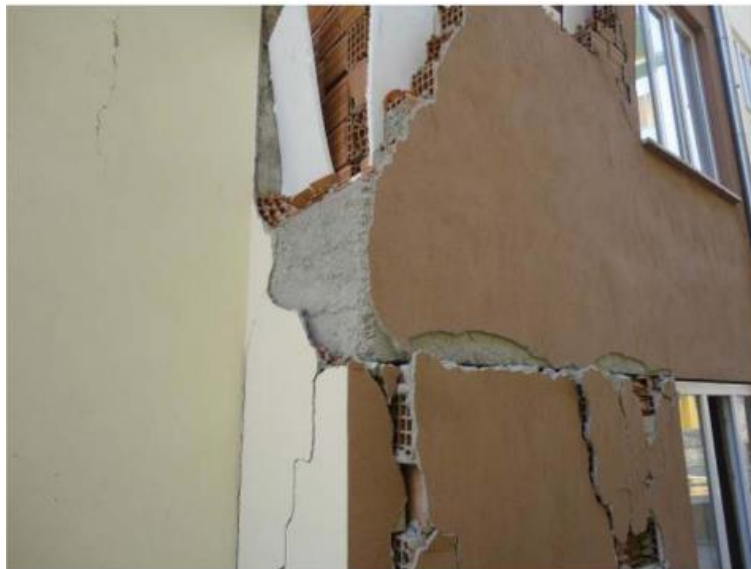
Figure 3. Failure to the multilayered infill wall and insulation inside [7].
