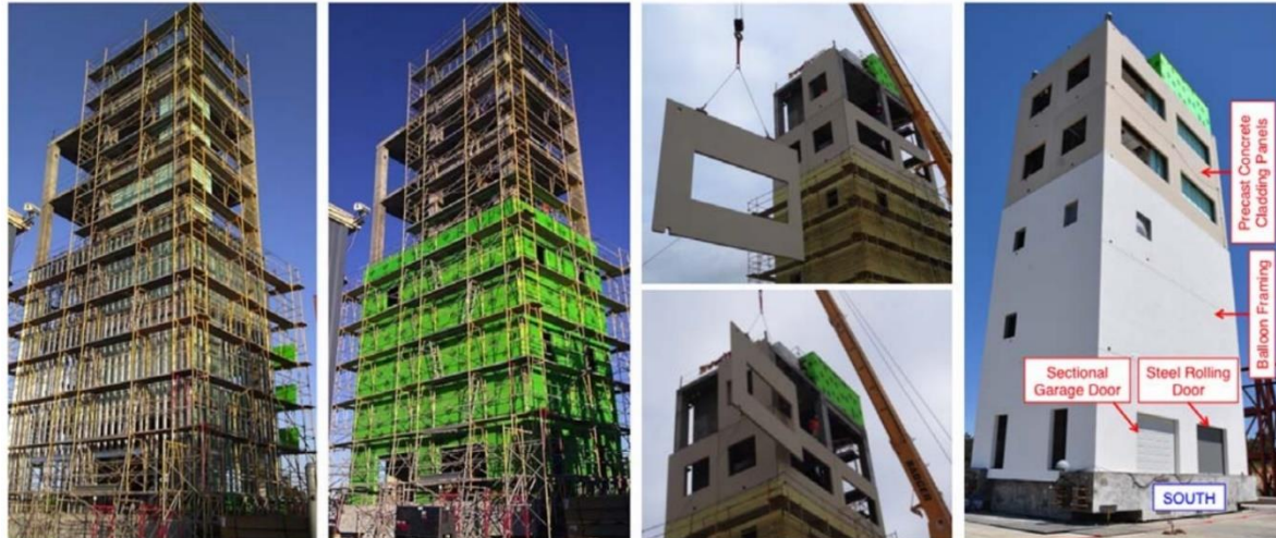
Figure 11. Full Scaled Five storey Building equipped with NSE's tested on Shake Table Tests [38].
