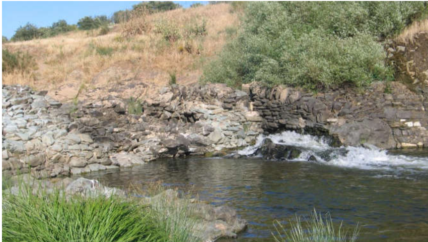
Figure 5. Water mill weirs made of stones, fitted perpendicularly to the flow of water, with the thickest part facing the outside of the construction (Guadiana River, Portugal) (Photo, Manuela Morais).
