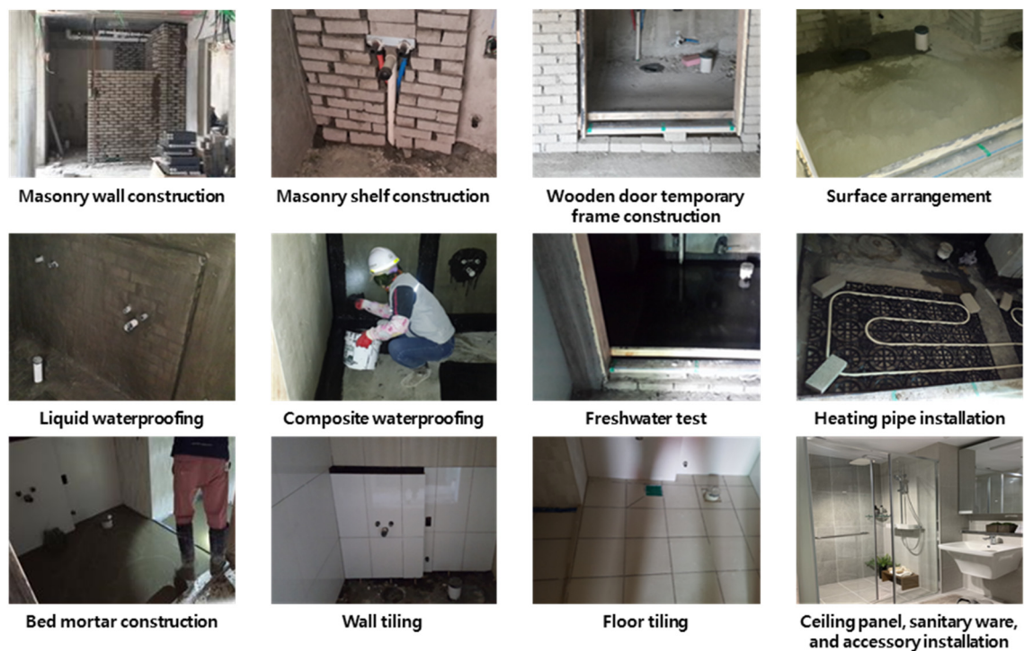
Figure 4. Wet bathroom construction sequence.
