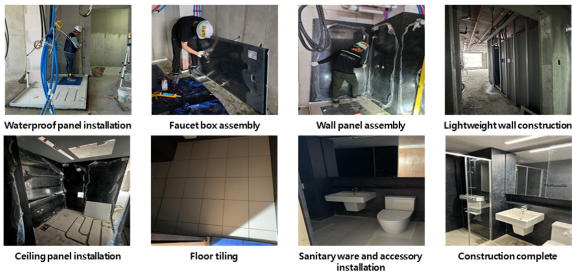
Figure 5. Modular bathroom construction sequence.
