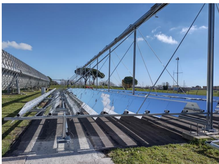
Figure 3. Linear Fresnel plant located at the ENEA Casaccia Research Centre (Rome).
