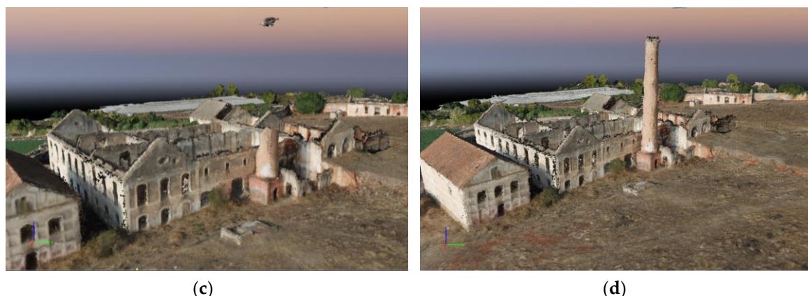
Figure 6. Dense point-cloud model of the San Joaquín sugar mill: (a) 12.5%, (b) 25%, (c) 50%, and (d) 100% of the acquired images.
