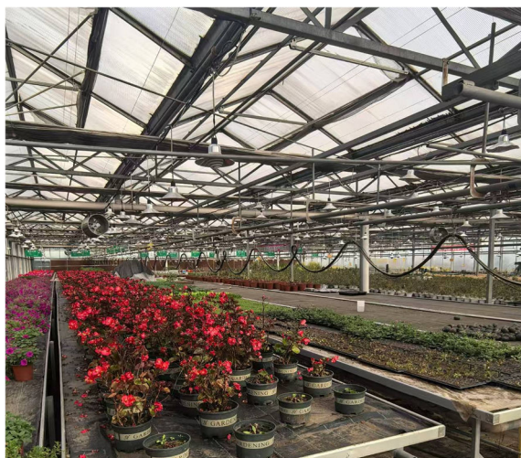
Figure 1. Supplementary Lighting System Inside the Greenhouse.
