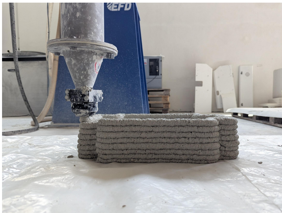
Figure 6. Robotic extrusion of a discrete block.
