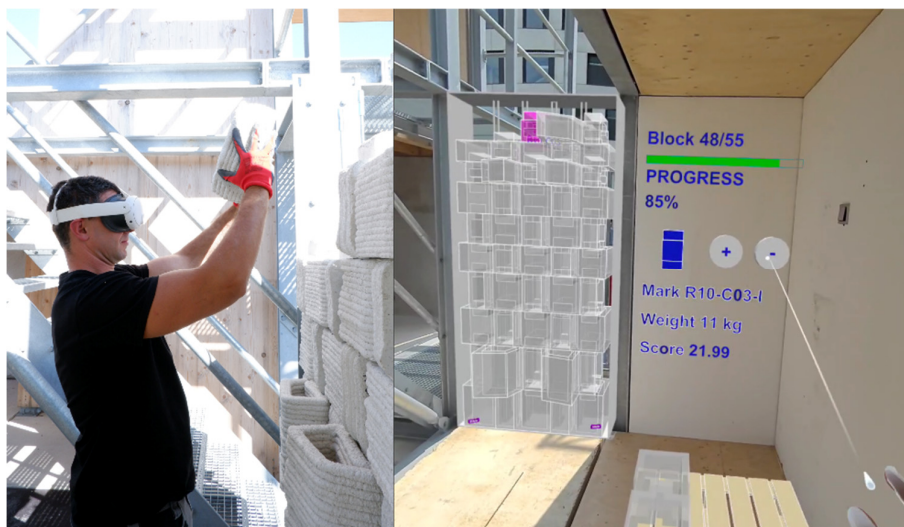
Figure 10. Assembly process using Meta Quest headset and Fologram.
