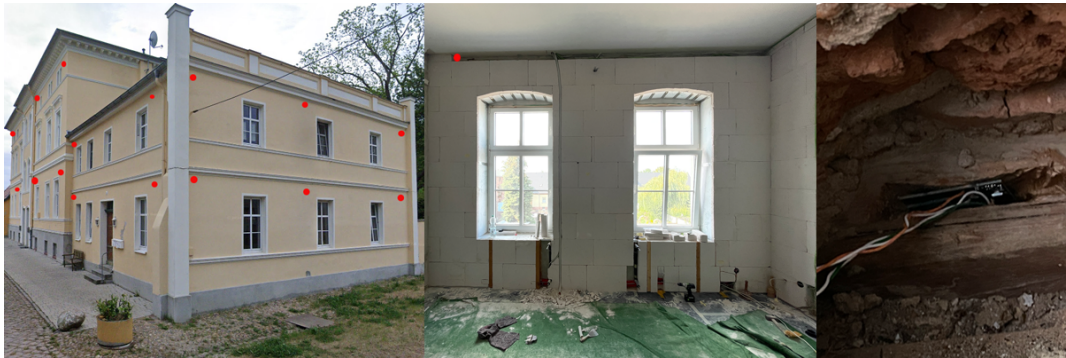
Figure 1. Positioning of sensors in room corners in a historic manor house from the Wilhelminian period, adapted from Finn E. Schmid-Bonde, Fachhochschule Potsdam.
