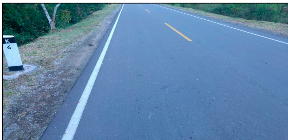
Figure 3. Surface condition of pavement applying nanotechnology. This image shows a section of road that has been improved using nanotechnology in the bituminous layers and stabilized bases. The results of the Pavement Condition Index (PCI) assessments over a three-year period demonstrate that these improvements maintain a "Very Good" condition.
