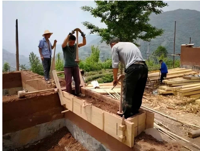
Figure 4. The traditional rammed earth wall formwork still in use in the village(Authors).
