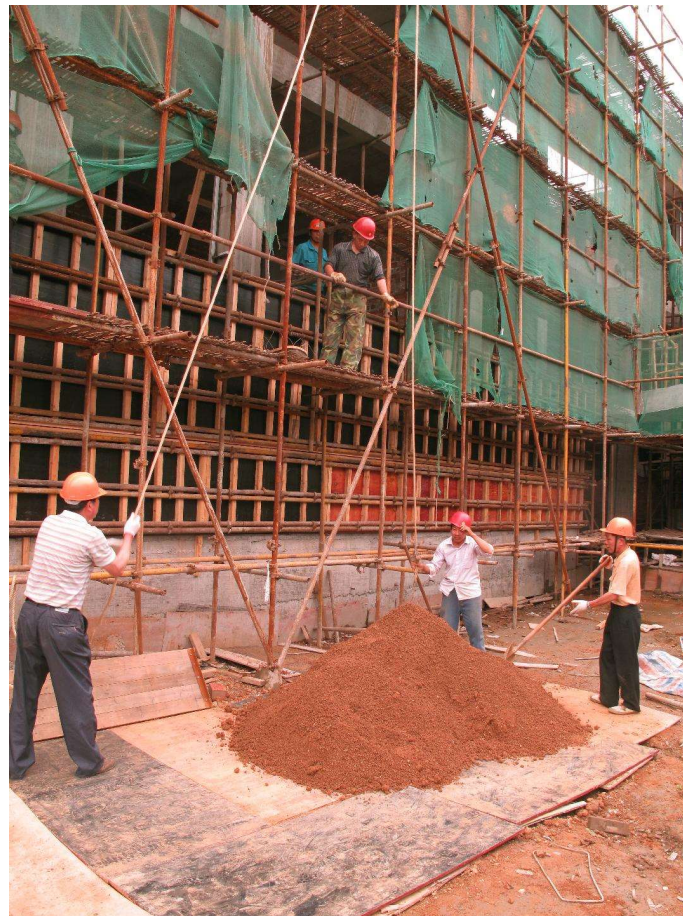
Figure 3. A rammed earth wall formwork technique akin to concrete pouring methods(Authors).
