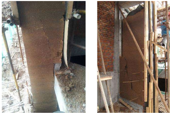
Figure 8. The wall has developed an outward tilt, leading to a large crack(Authors).
