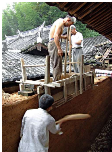
Figure 5. In the traditional practice, specialized craftsmen patted down the finished rammed walls(Authors).
