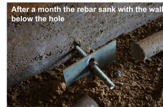
Figure 15. tructural joints used in modern construction systems to prevent outward tilting of earth walls(Authors).
