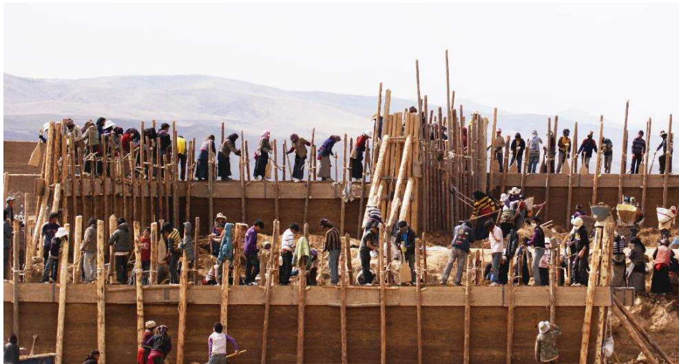
Figure 18. A scene of villagers in the Tibetan region engaged in the rammed earth construction process[12].
