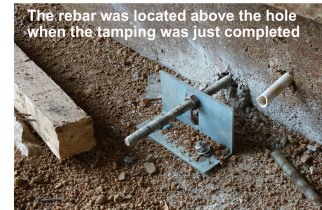
After a month the rebar sank with the wall below the hole
