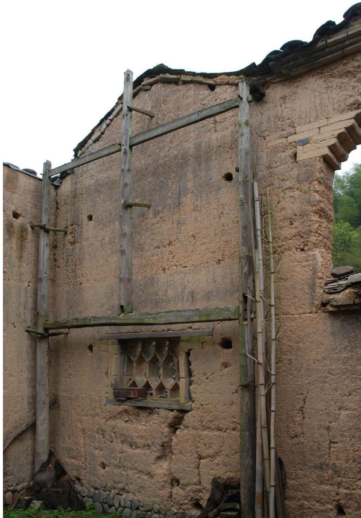
Figure 13. Connection between traditional rammed earth walls and the main wood structure(Authors).
