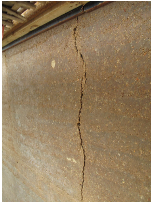
Figure 9. The wall exhibits vertical fine cracks(Authors).
