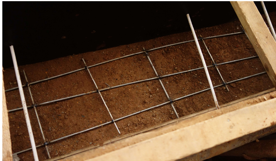
When rammed to the floor level, an additional layer of rebar lattice is added to the earth wall, through which the wall is pulled
