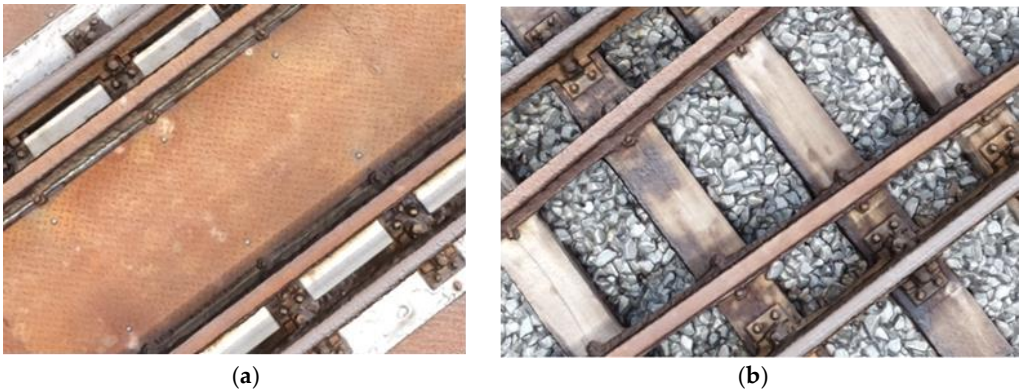
Figure 20. Detail view of the railway structure Agisoft 3D model: (a) on the bridge; (b) at the approaches to the bridge..
