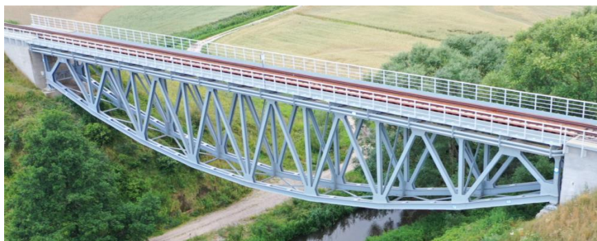
Figure 2. Overall view of the Niestepowo Bridge.
