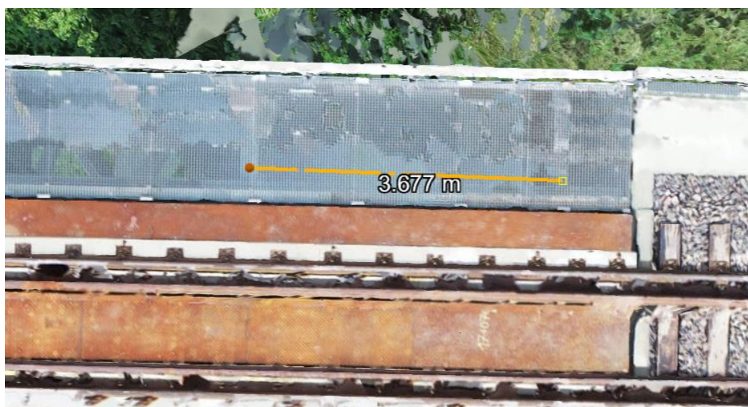
Figure 18. Bentley 3D model measurement of the crossbeams spacing.
