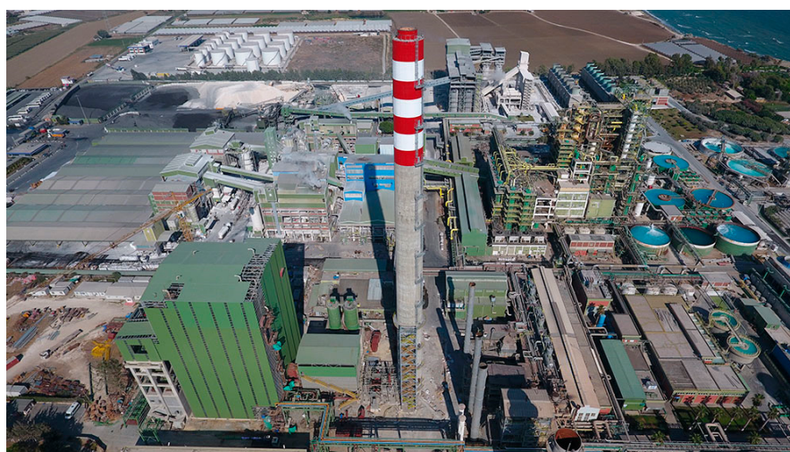
Figure 1. General view of the Mersin Soda Factory chimney [28].
