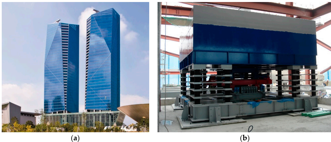
Figure 1. Benchmark structure: (a) Overview of the Posco E&C Tower in Songdo, South Korea; (b) 160-ton tuned mass damper.
