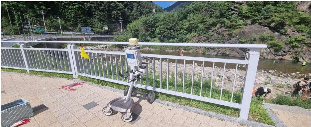
Figure 12. Bridge Measurement Location (V3, Landside) in Chilrangi Valley.
