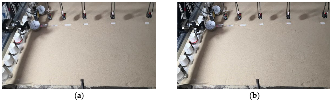
Figure 27. Surface photos of R3 for different excavation depths: (a) The excavation depth is 70 cm; (b) The excavation depth is 80 cm.
