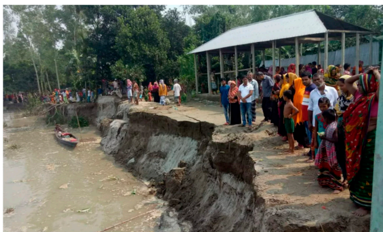
Figure 1. Flood defence system collapsed a year after construction in Bangladesh, Sirajganj (Image from DhakaTribune [6]).
